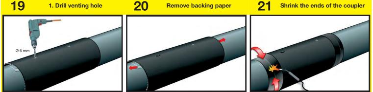
Now slide the coupler over and align using the two centring marks Drill first venting hole with a 6mm diameter. Remove backing paper of the butyl rubber sealing tape on both sides.
