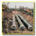
All **isoplus**-products might be used for different applications such as heating, sanitary, steam, cooling pipes, oil, chemical and foodstuff industry etc. and temperatures at least according to EN 253. Perfect welding engineering within the steel and PE area guarantee solid products with the necessary operational reliability.
